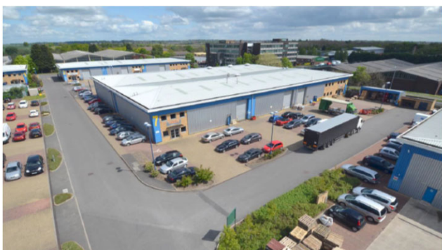
Northampton, IO Centre, Lodge Farm Industrial Estate
