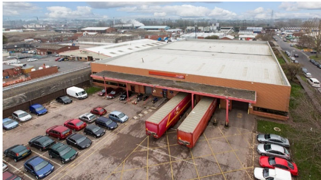
Exeter, 13 Trusham Road, Marsh Barton Industrial Estate
