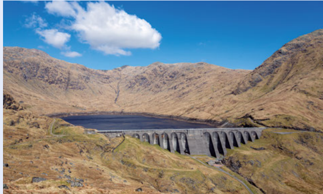
Cruachan 440MW capacity
