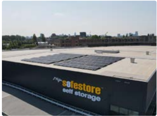
Rotterdam with a new PV Cell system.
