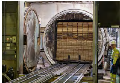
Reactor in Arnhem plant
