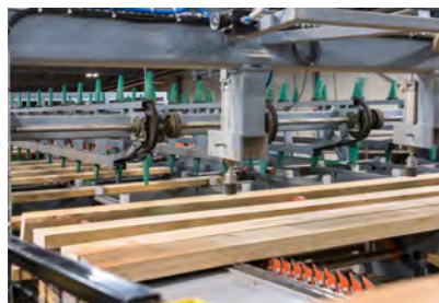
The new wood stacking process machinery at the Arnhem plant
