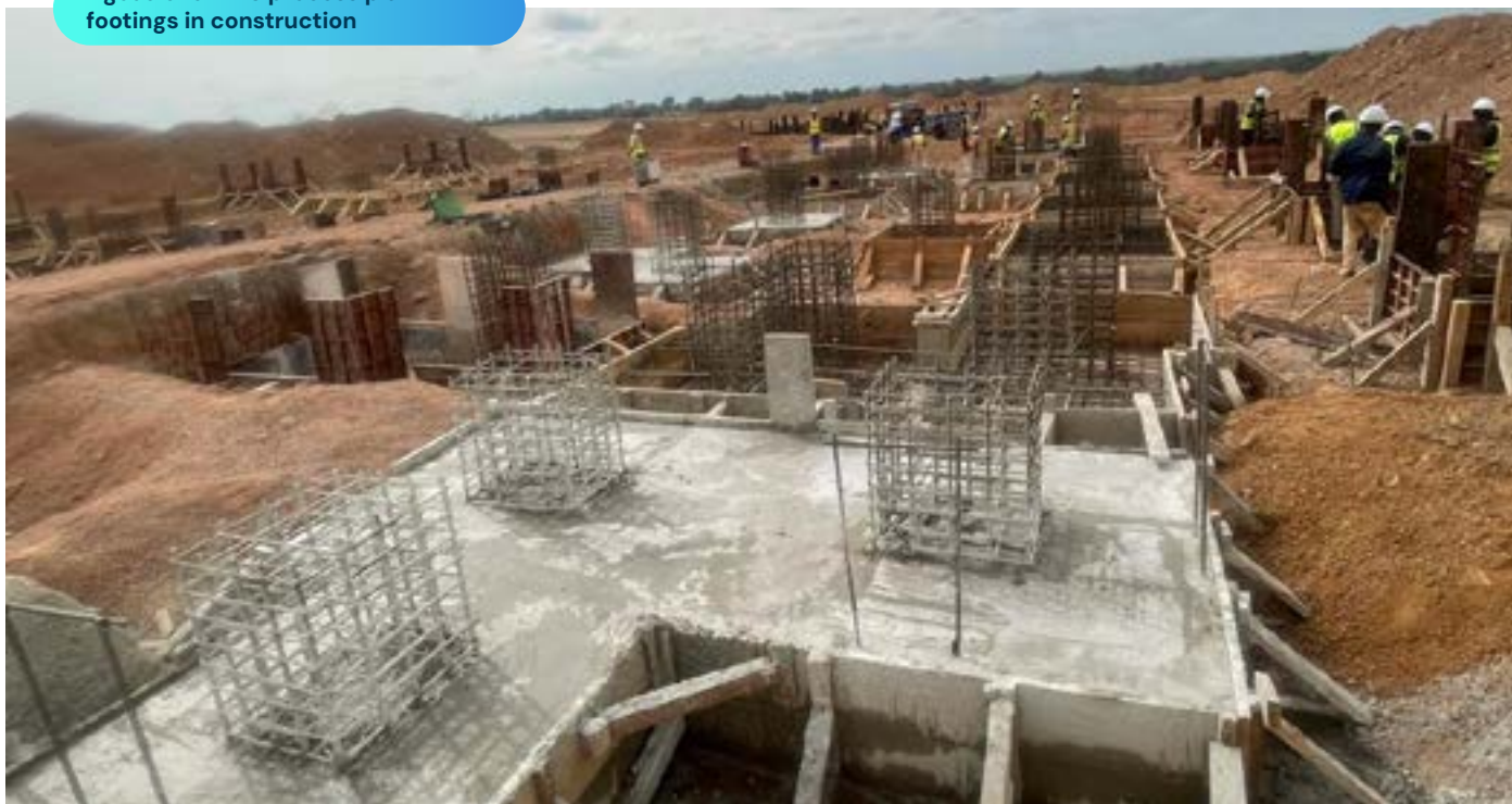
Ngoualana DMS process plant footings in construction
