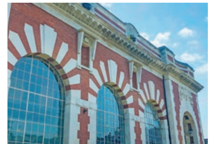
21,268 sq ft ground floor unit let to Metropolis
