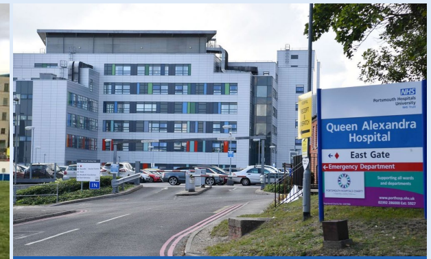
Queen Alexandra Hospital, Portsmouth HV Infrastructure upgrade Status: *PCSA £23k Project Value: £6m
