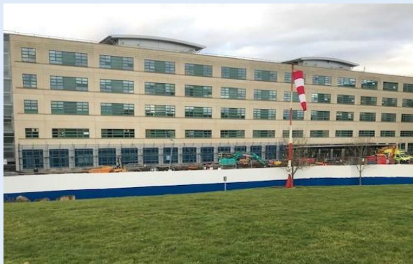
Great Western Infirmary, Swindon Status: On Site summer 2023 Project Value: £6m
