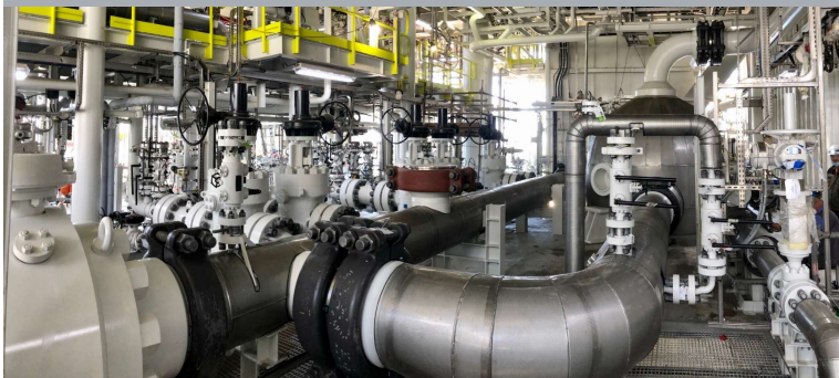
Manifold and separator
