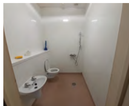
Fully accessible bathroom refurbished to doc M building regulations.
