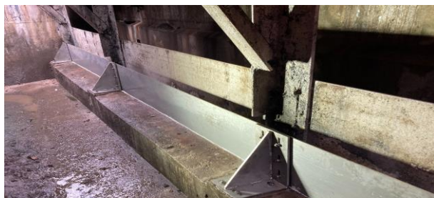
Weir raise completed at Ironville storm overflow
