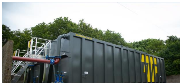
Submerged Aerated Filtration units installed at Hurley
