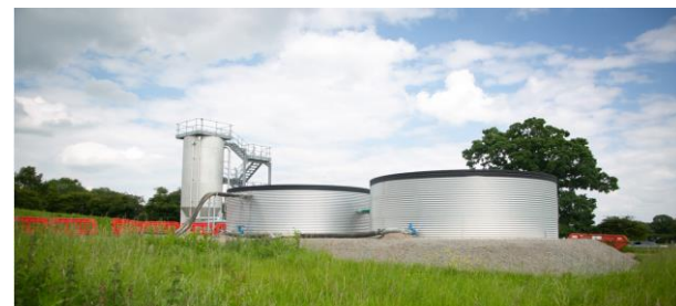
Storm tanks installed at Braunston
